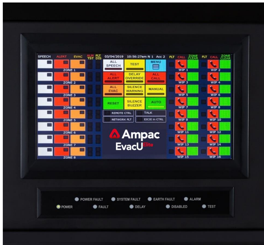
Figure 4-11 Main GUI and LED membrane
