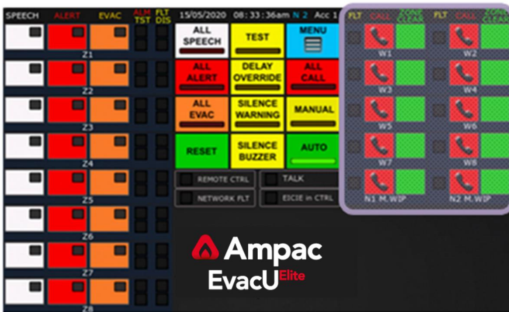
Figure 5-5 Front control panel with the individual EIS controls and indicators highlighted.
