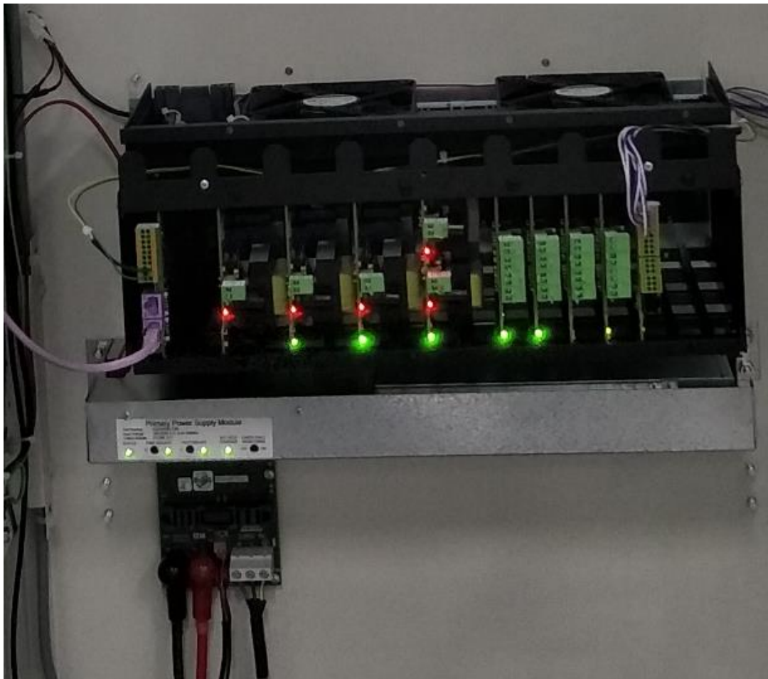
Figure 4-10 Power supply - showing the primary power supply module.
